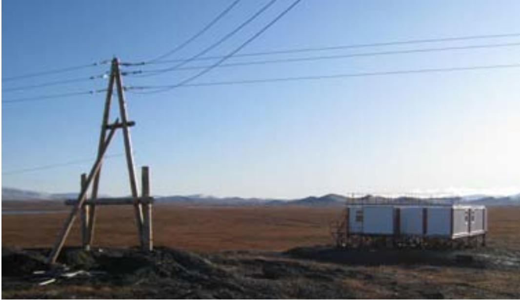
Figure 4.3 Exterior of new Central Observatory and Weather Building in September 2009
