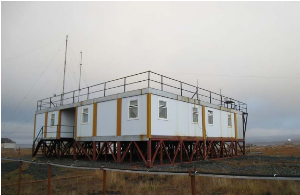
Figure 4.1 Exterior of Central Observatory and Weather Building
