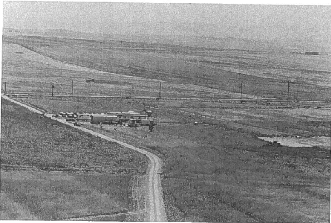
Figure 24.2. Temporary building and launch areas for balloons and aircraft.
