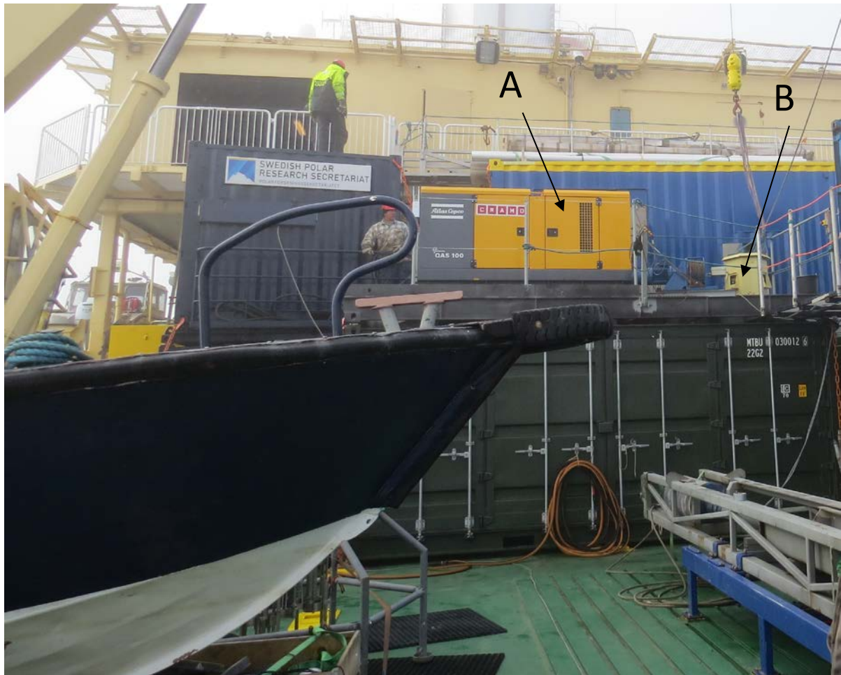
Figure GM-14: Generator (A) and transformer (B) of electromagnetic field
