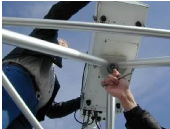
Figure 3-8. Securing the Profiling Radiometer with the T bolt
