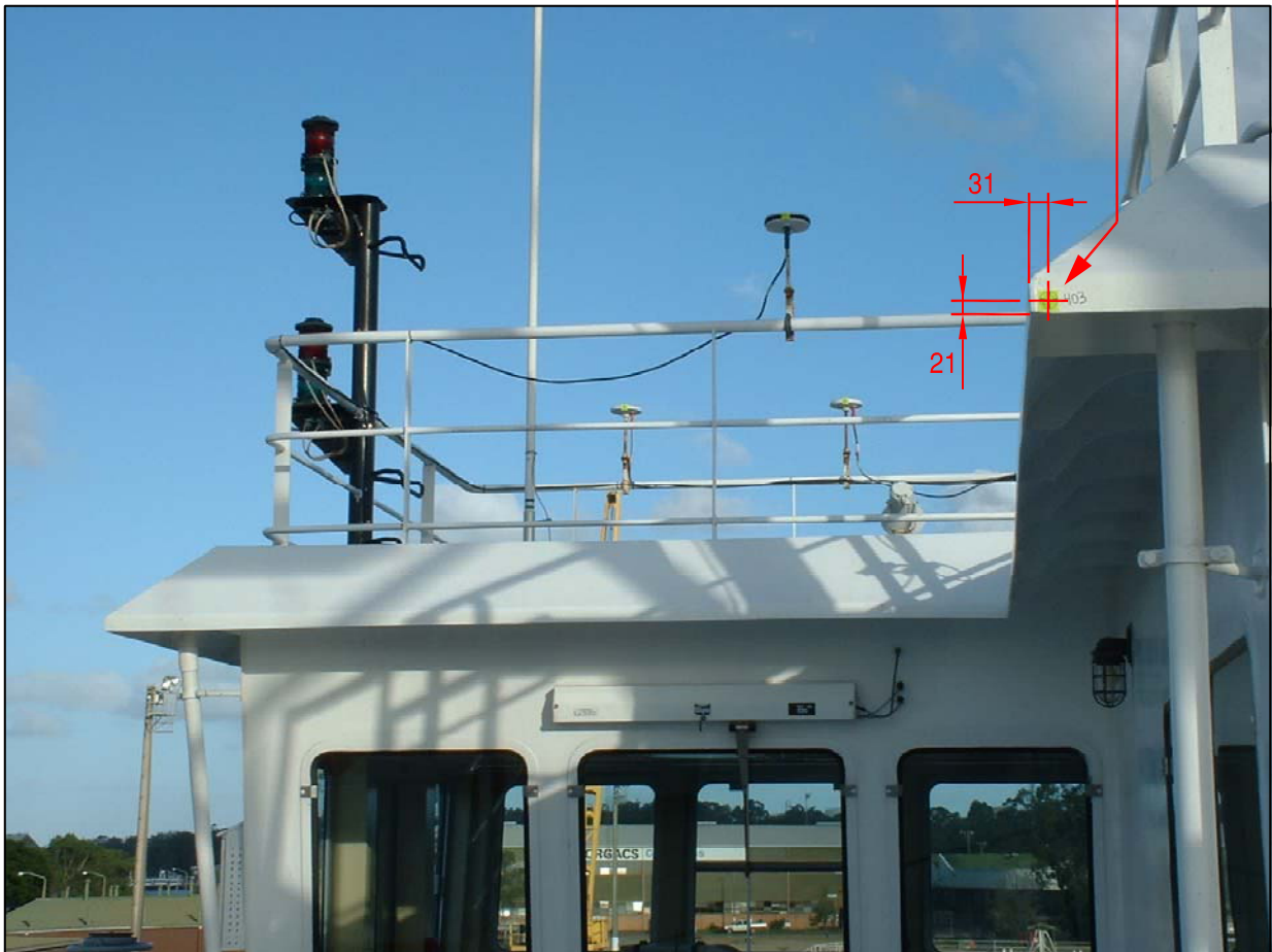
AFT SIDE WHEELHOUSE ROOF (LOOKING FWD)
