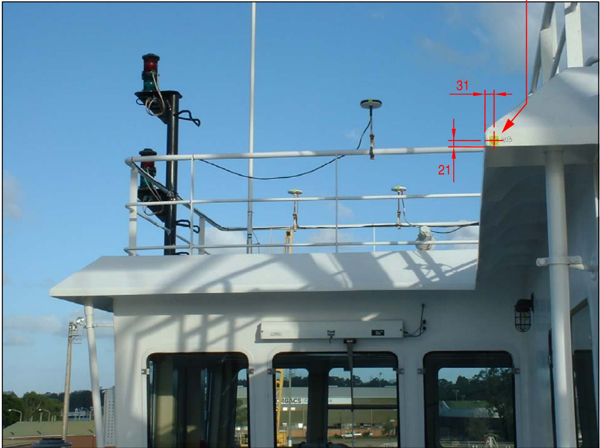
AFT SIDE WHEELHOUSE ROOF (LOOKING FWD)
