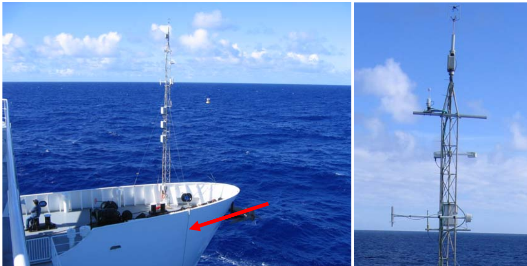
Figure 2. Left: Flux tower deployed at the bow of the portside pontoon. The sea surface thermistor, i.e. 'sea snake', can be seen on the inboard side of the pontoon (red arrow). Right: Close-up view of the tower and its instruments
