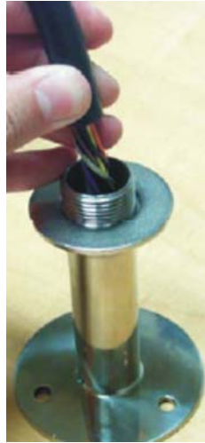
Figure 1-15. Running cable through the pole base
